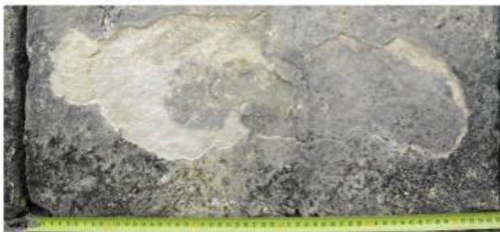
Figure WP2.9 - Evolution of the alteration of the surface of a stone (lithofacies C according to WP1 determination: grey massive limestone) on the West wall of Volubilis Basilica (Volubilis Morocco) in presence of soluble salts from 2006 to 2008.
