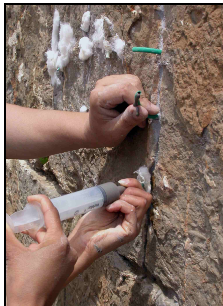
Figure WP3.6 - Reinforcement of small scales by injection of home-made mortar using a syringe (Septimian temple Djemila, Algeria).
